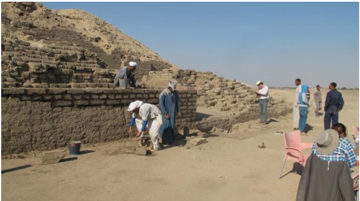
Fig. 5 A layer of geotextile mesh was added between the modern and ancient courses in the “South Palace” restoration.
