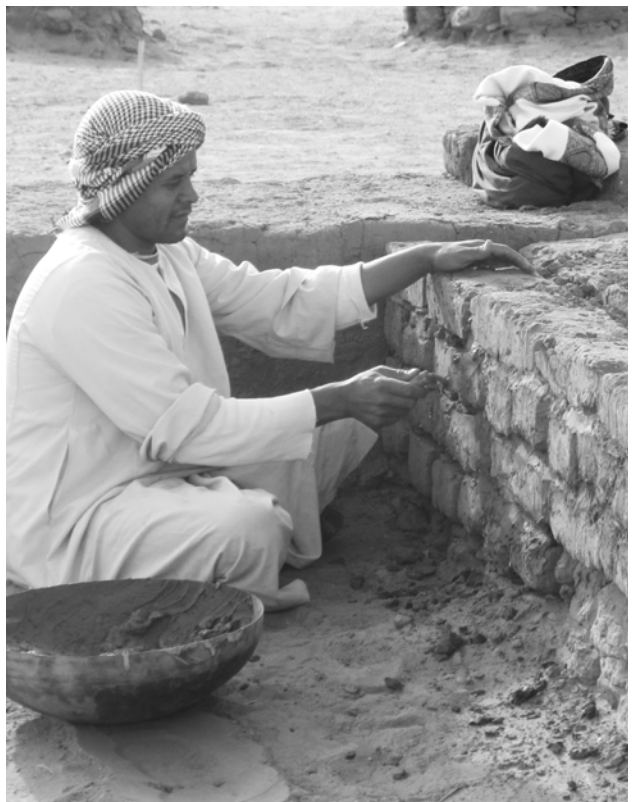
Pointing the new mud bricks
