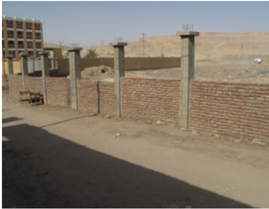
Barrier wall under construction
