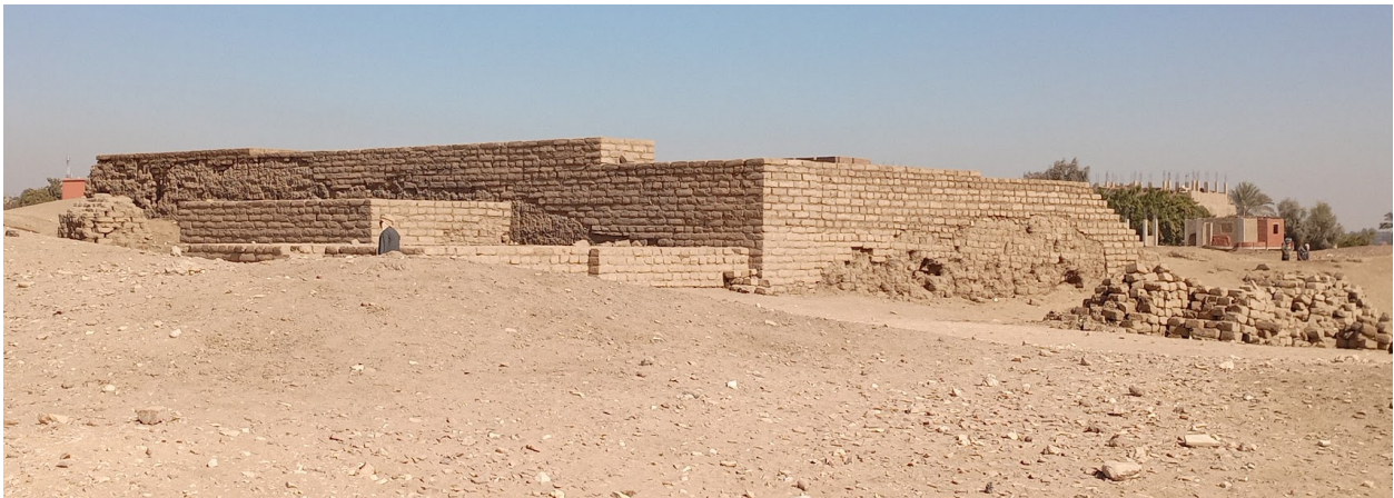
Fig. 2 Capping the casemate foundations of the North Palace in 2023. (Photograph by Peter Lacovara)
