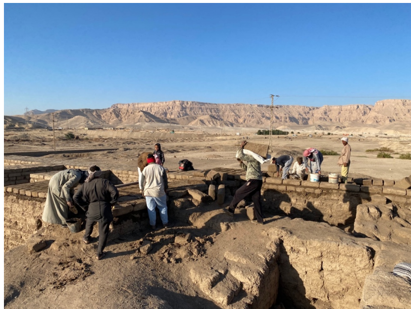
Figure 4: Restoration work at the North Palace.
